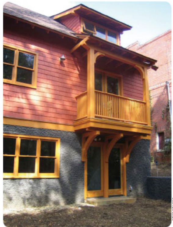
Well-insulated, precast concrete basement walls contribute to the Beili home's energy efficiency.
