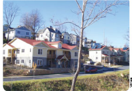
Prospect Terrace, an affordable green development, was the pilot project for the NC HealthyBuilt Homes Program.
